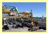
Engineered Bidwell working as a gantry crane
